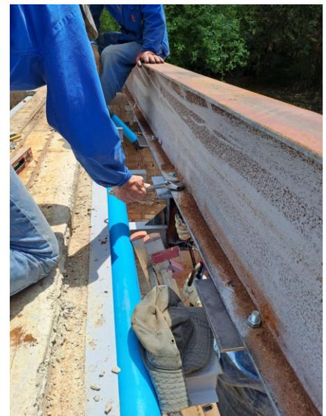
Off loading and getting the beams and support brackets in-place (with specialised tools!), aligning and welding.
