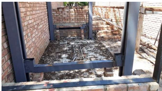
Lift stanchions now in place in the new storage.
