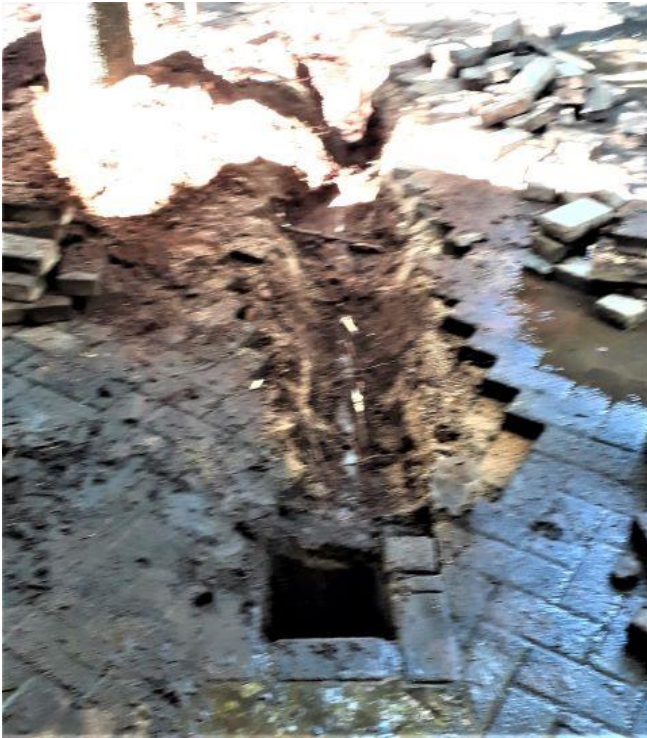
Excavating the drainpipe
