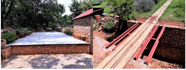
air supported by the generous use of reinforcement in the concrete. A steel structure has been fabricated from steel in our stock to form a new bridge to support and carry the track over the culvert. We are hoping the project will be completed for March Track Day.
