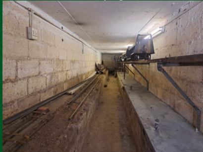
Some serious work going into storage tunnel 1 & 2. The Tuesday gang modifying the track support for storage area.
