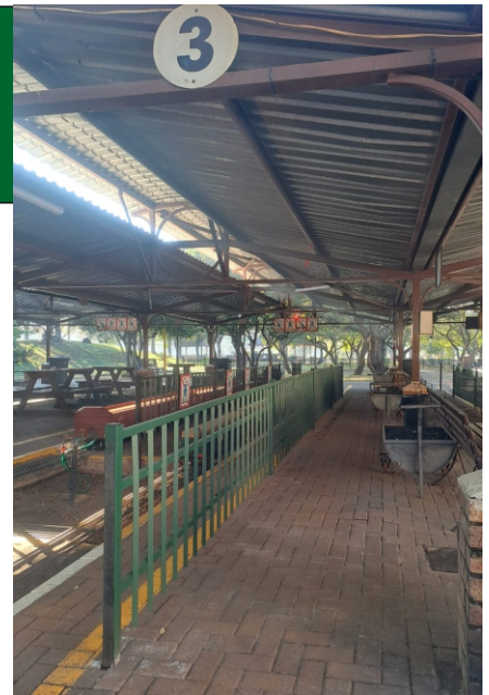
Palisades for platform 3 done, with 4 in progress. This assist greatly to improve passenger flow during boarding and disembarking.
