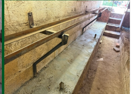
Some serious work going into storage tunnel 1 & 2. The Tuesday gang modifying the track support for storage area.
