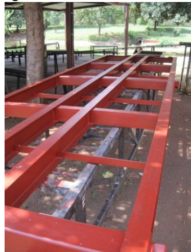
Above right shows one of the two completed spans to go each side of the bridge centre, now ready to be fitted.
