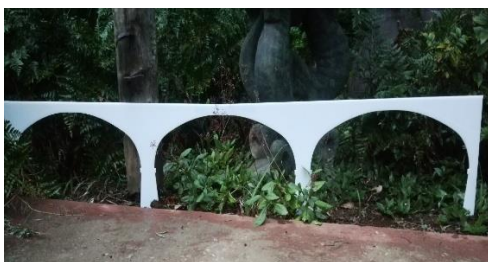
Side panel for the Fountains Valley bridge to be cast out of cement.
